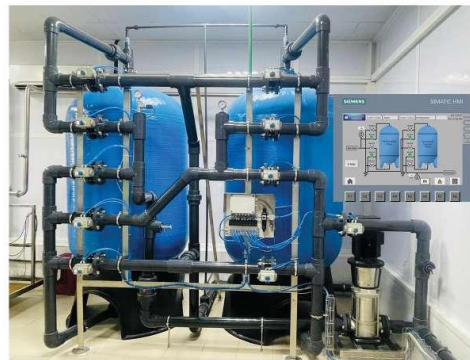
Automatic Pre Filtration units operated from HMI
