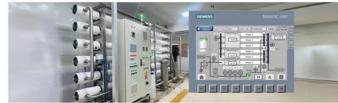
PLC Based Remotely Monitored and Controlled SWRO Plant
