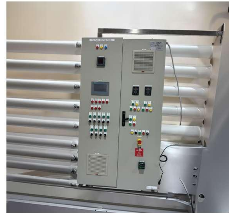
RO Plant Control Panel
